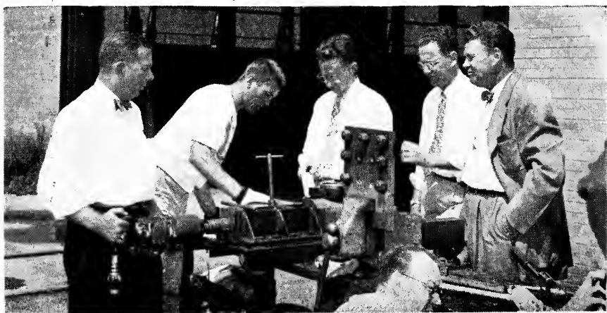
Fig. 1—Calibrating an impact wrench with a hydraulic calibrator before tightening experimental high-strength bolts.
